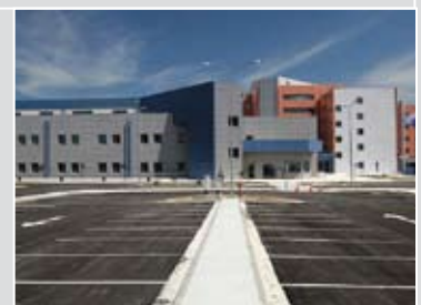
General Hospital of Kavala, Greece
